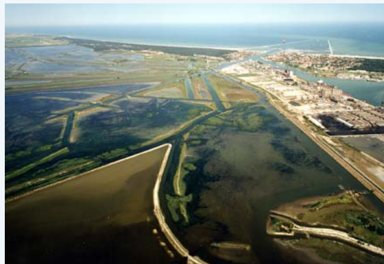
Fig. 1. The Pialassa Baiona lagoon and the adjoining harbour/industrial area (by Biserni, 1999).
